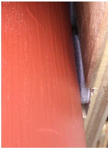
Figure 5: Pads to allow movement of tube
