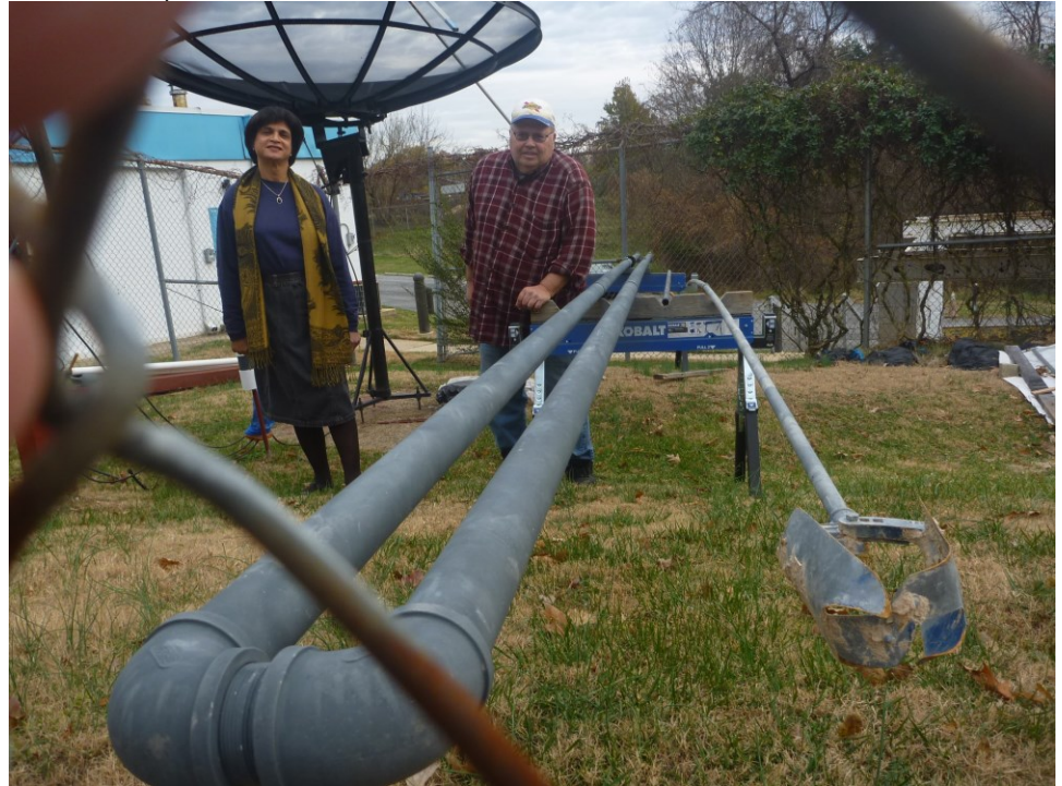
Sarah Brown and Duane Bratlie alongside a 30-foot U-shaped pipe and the auger for digging the hole the pipe will go in.
