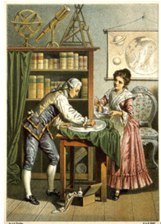
Image: William and Caroline Herschel polishing a telescope lens or mirror. (Lithograph, 1896 CE)
